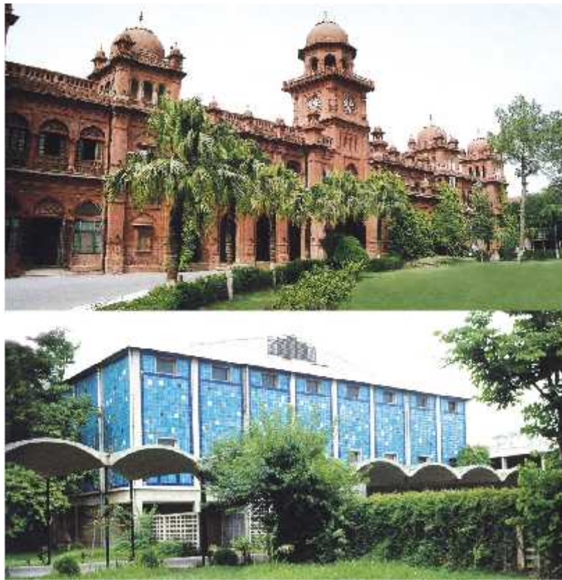
Punjab University Old Campus Building and Faisal Auditorium in New Campus
